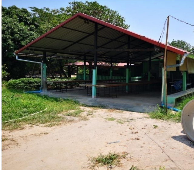
Rainfall harvesting system
